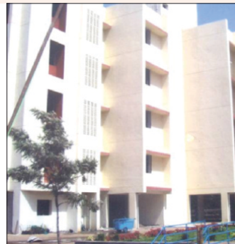
Pune, Ph-II : 148 DUs Completion Year : December, 2008
