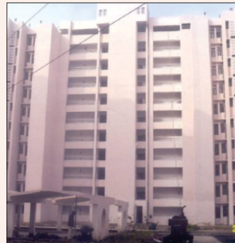
Mohali, Ph-I : 603 DUs Completion Year : April, 2013
