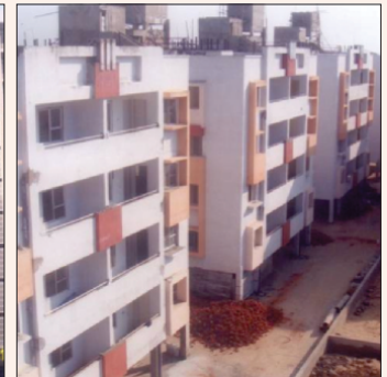
Bhubaneswar, Ph-I : 256 DUs Completion Year : January, 2013
