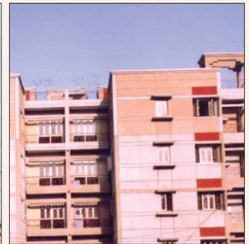
Gurgaon, Ph-I : 1088 DUs Completion Year : July, 1999
