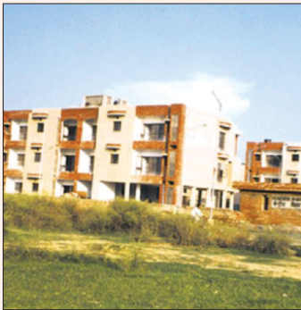
Chandigarh : 305 DUs Completion Year : May, 2000
